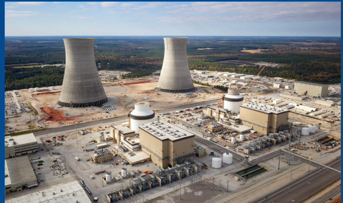
Plant Vogtle Unit 3&4 Nov. 2022
