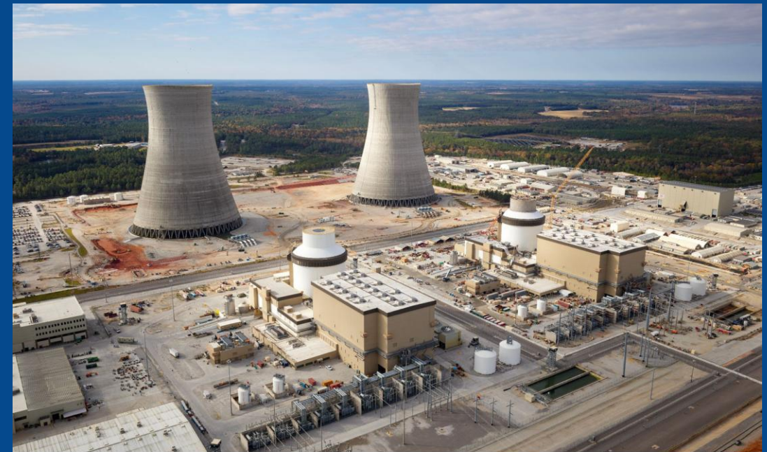
Plant Vogtle Unit 3&4 Nov. 2022
