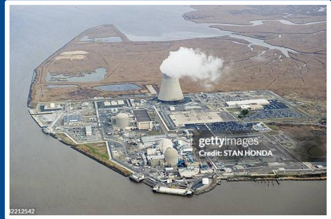
Hope Creek Nuclear Generating Station, NJ
